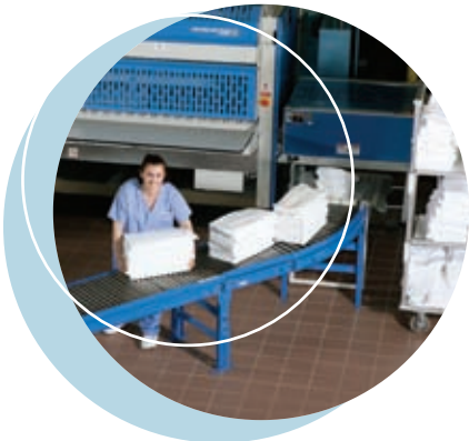
The new conveyor system cuts down on travel for staff and reduces the number of carts on the plant floor, increasing productivity.
